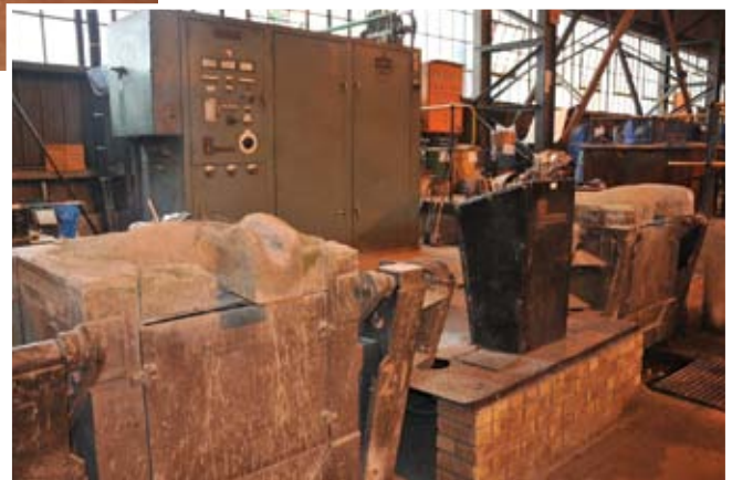
The foundry has two 500 kilogram furnaces, a 5-ton an hour Omega mixer that has been fitted with an auto blend unit and they are currently installing an Omega sand reclamation plant
