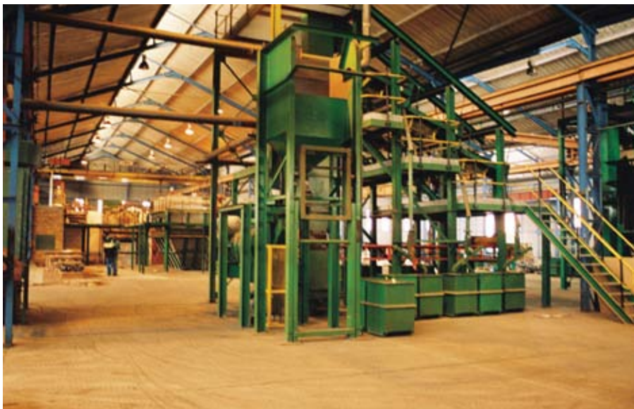
Dedicated product processing lines consisting of retrieval, screening, crushing, classifying and packaging, exist for the different products produced by the company
