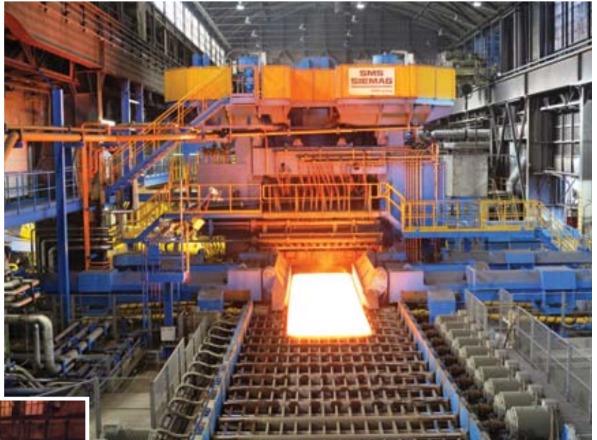
The inside of a steel mill
