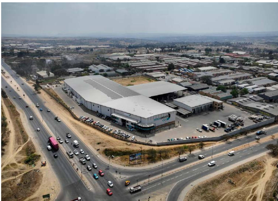
Hitech-Gregfor’s new facility in Kya Sands, Gauteng
