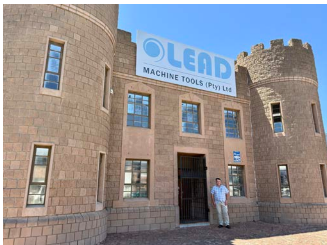
Mark Burn, Lead Machine Tools' General Manager stands outside Lead Machine Tools' new building that the company has purchased and moved into. Fittingly, the building features a number of turrets as part of its architecture
